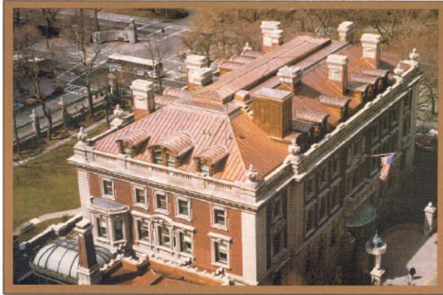
ROOFING CONTRACTOR: NHO CONTRACTING CO., PITTSBURGH, PA
